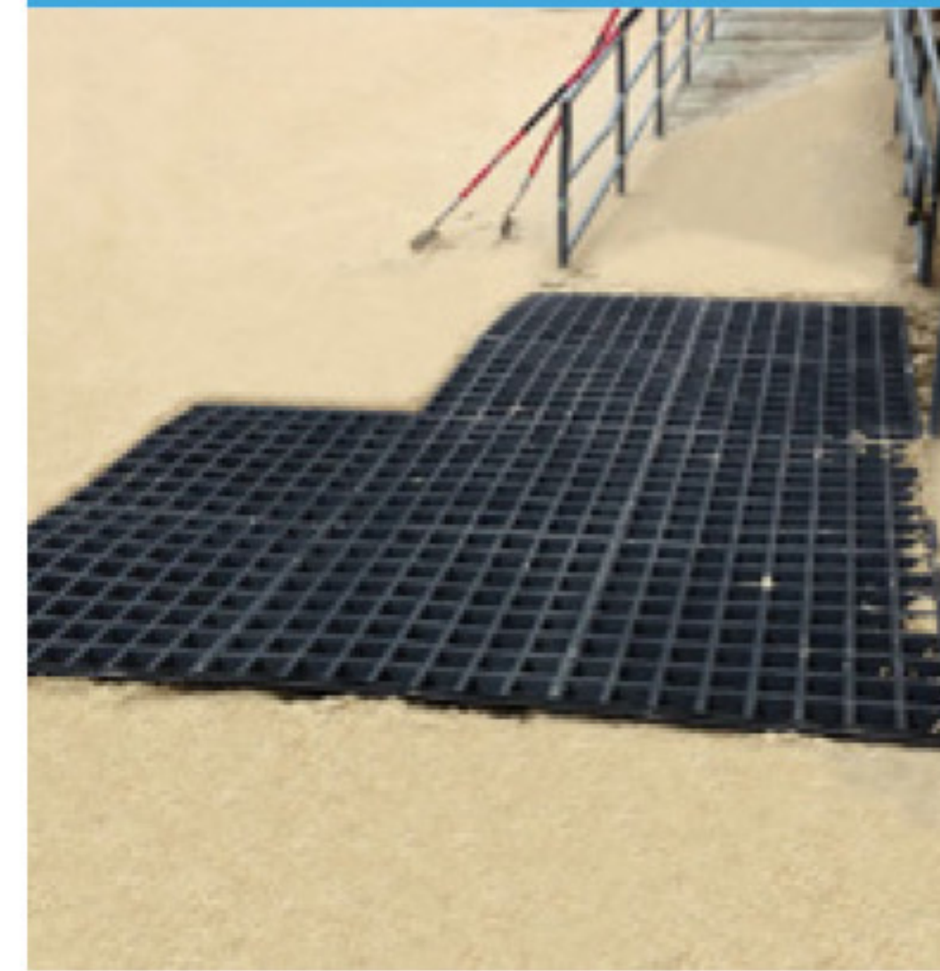
excavate 3" of sand
