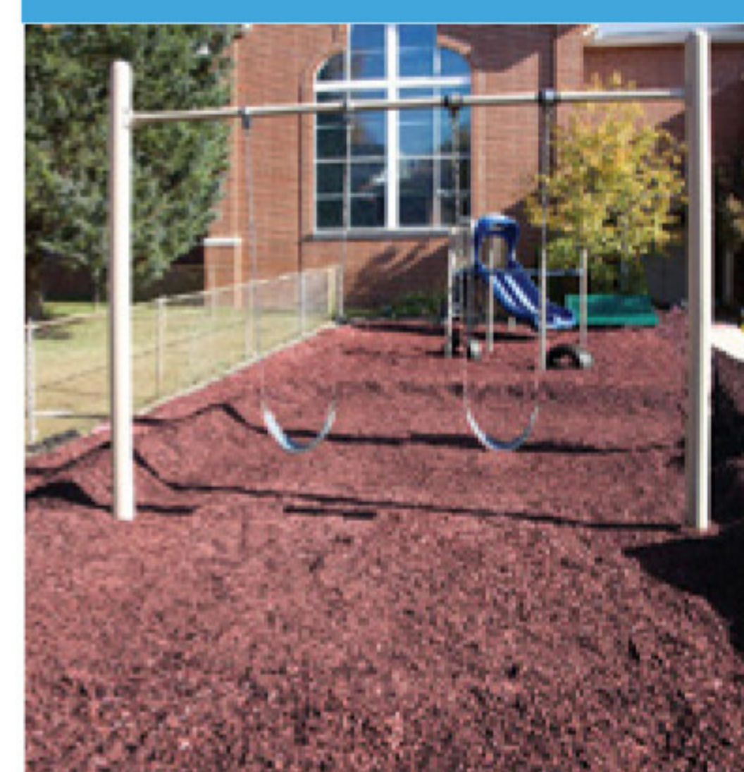
3" of mulch placed
