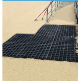
excavate 3" of sand
